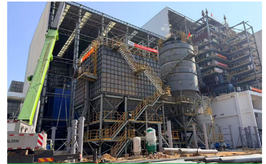
Construction site of the second phase of the Domestic Waste-to-Energy Power Plant
